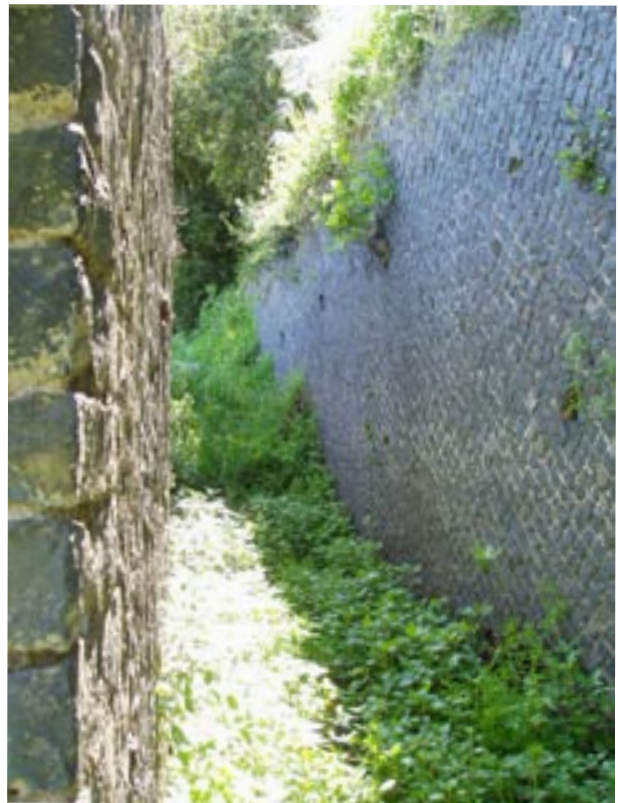
Fig. 7. View of the ramp (author's image).
