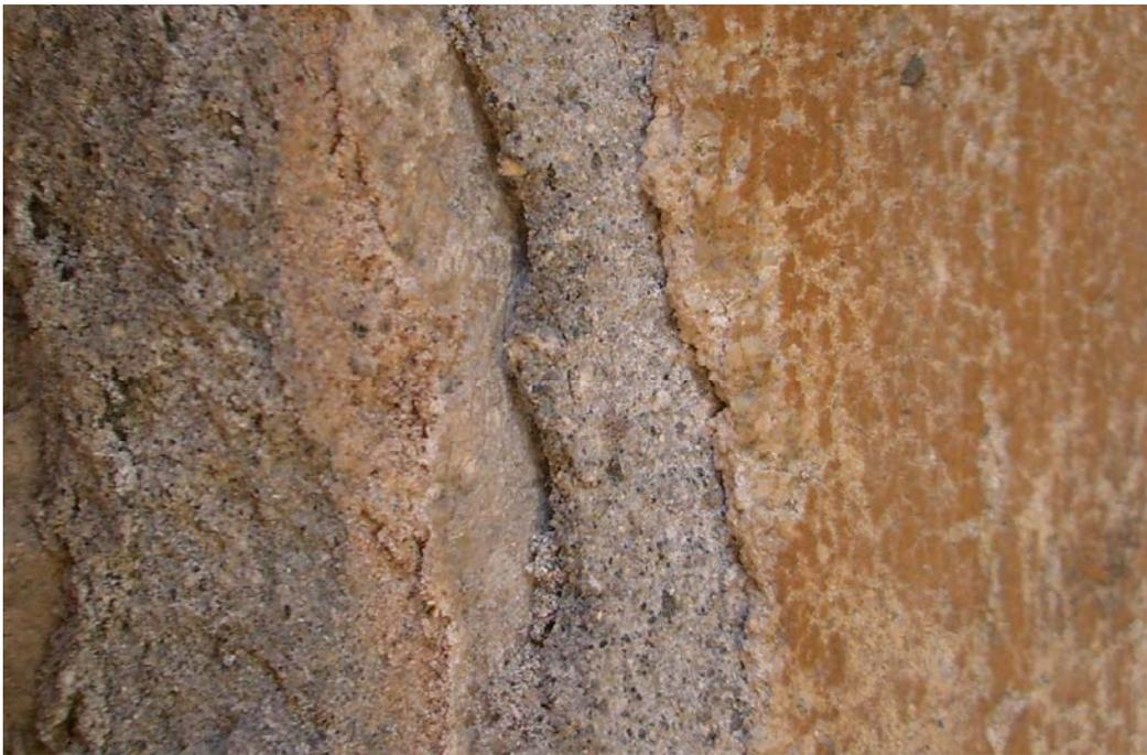
Fig. 6. *Above*: I 9 11 Casa di Amarantus. Plaster on the east wall in the bar area, room 2, containing crushed and reused materials, such as ceramics, glass and marble.
