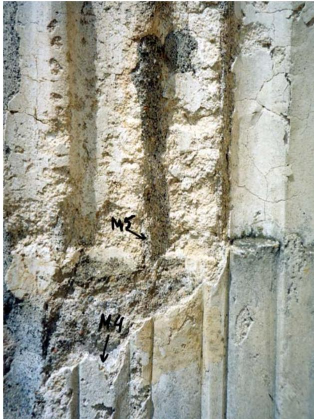
Fig. 49. Macellum. Sampling areas M4 and M5. The lower part of the pilaster has most probably been redecorated, due to earthquake damages.
